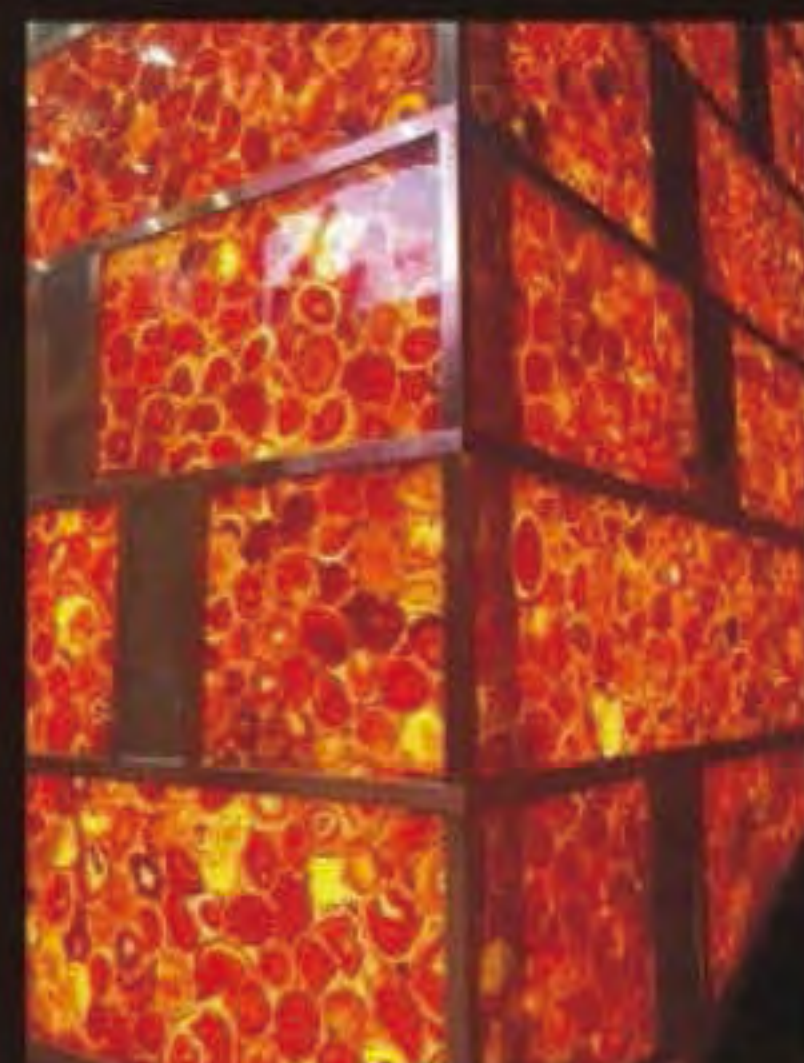
外立面-红玛瑙 External walls-red agate
